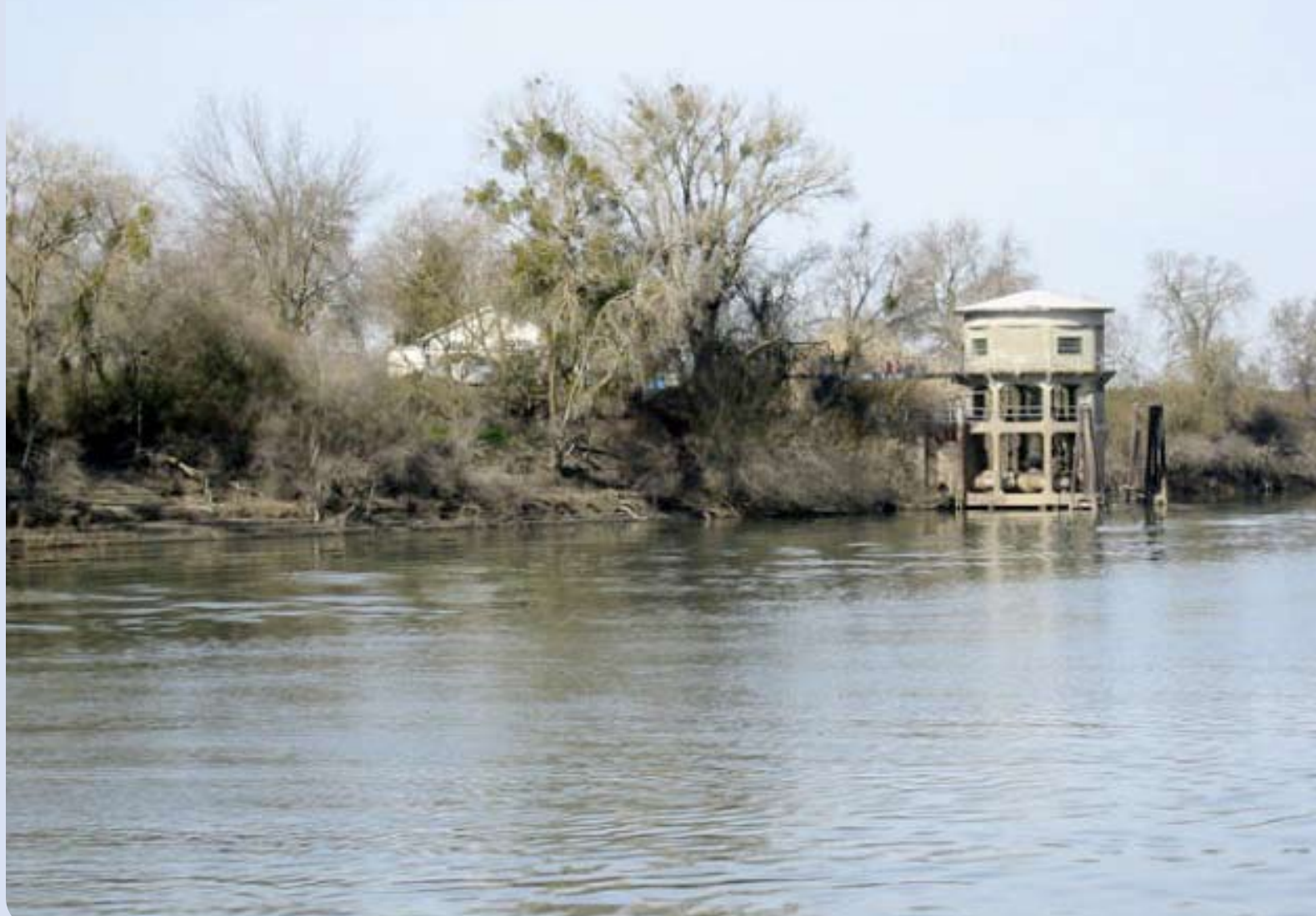
Existing Intake Structure - Built in 1920
