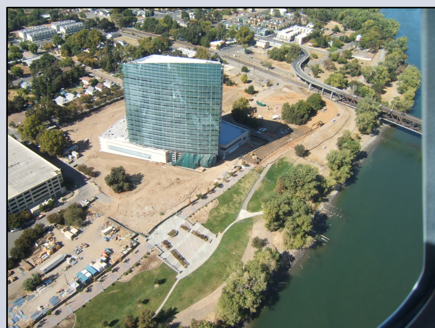
West Sacramento Levee Improvement Project I Street Bridge City of West Sacramento
