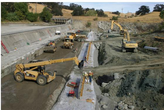
**Capay Dam Apron Repair Under Construction
