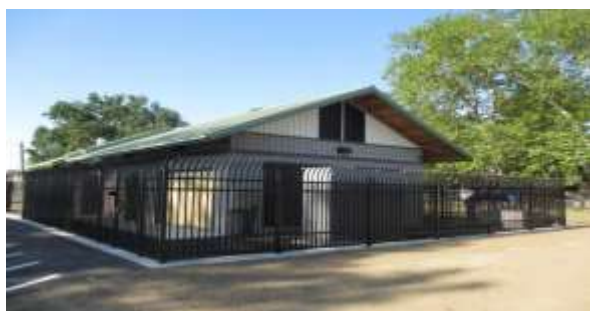
City of Woodland, Aquifer Storage & Recovery Project, Well #28
