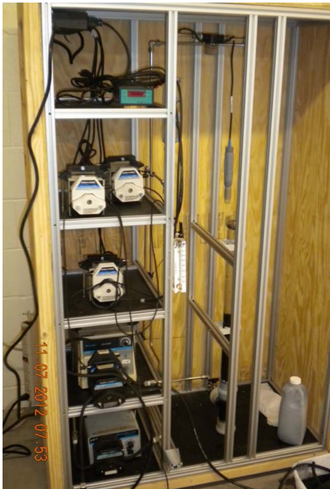
Photo #4: Pilot System
